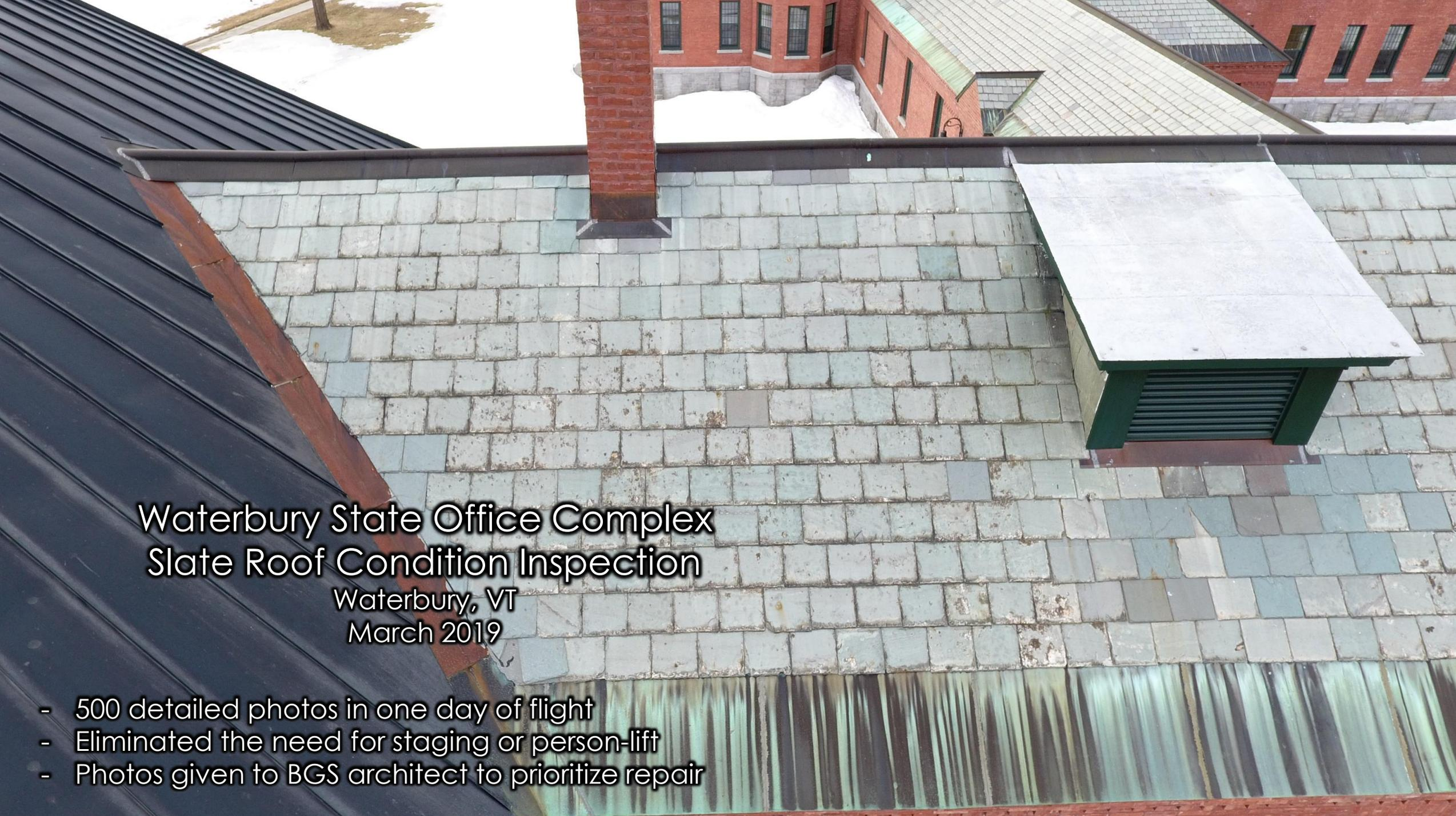
An aerial photograph of a slate roof. A brick chimney is visible in the upper center, and a green vent is on the right. The roof is covered in grey slate tiles, some showing signs of wear and discoloration. A dark metal roof is visible on the left side.
